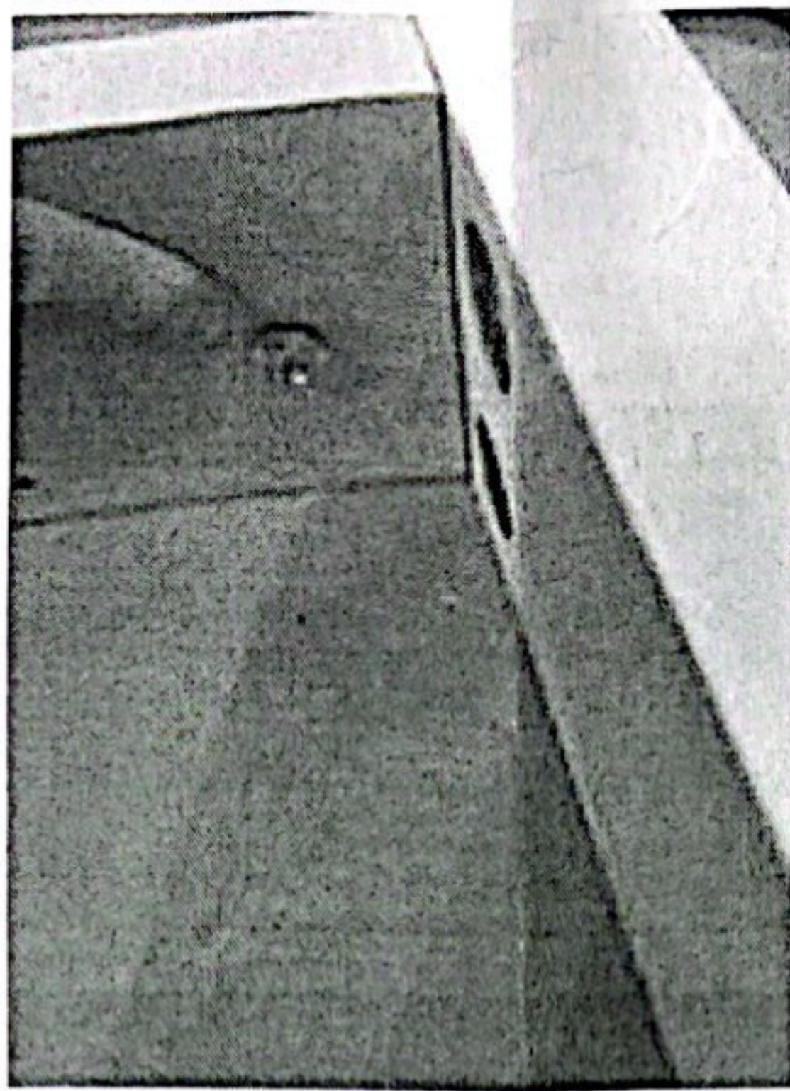
UNION BETWEEN SIDERAILS WITH INTERIOR FOOTBOARD
