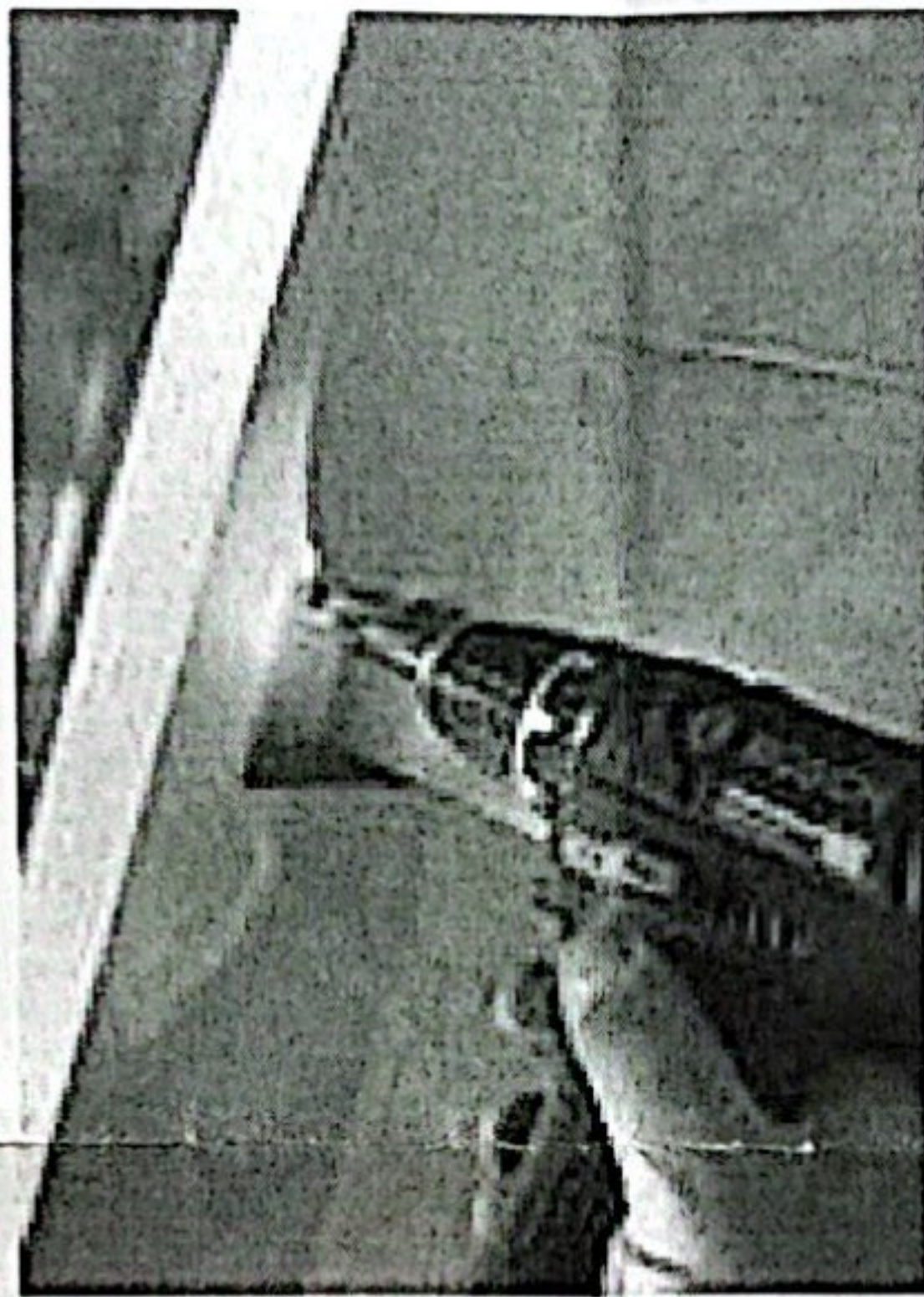
ASSEMBLY METALLIC CROSSBARS WITH SIDERAILS
